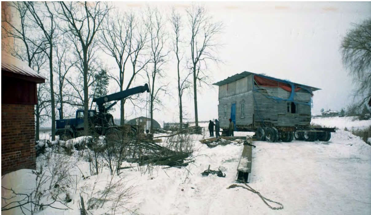
Figure 37 – The Norton Cabin was initially placed on wood supports closer to the back of the meadow, within the Study Area. This photo from November 1997 shows the cabin being moved to the site. A hoop house is visible in the background. Photo taken from The Brown Homestead collections, not available online.
